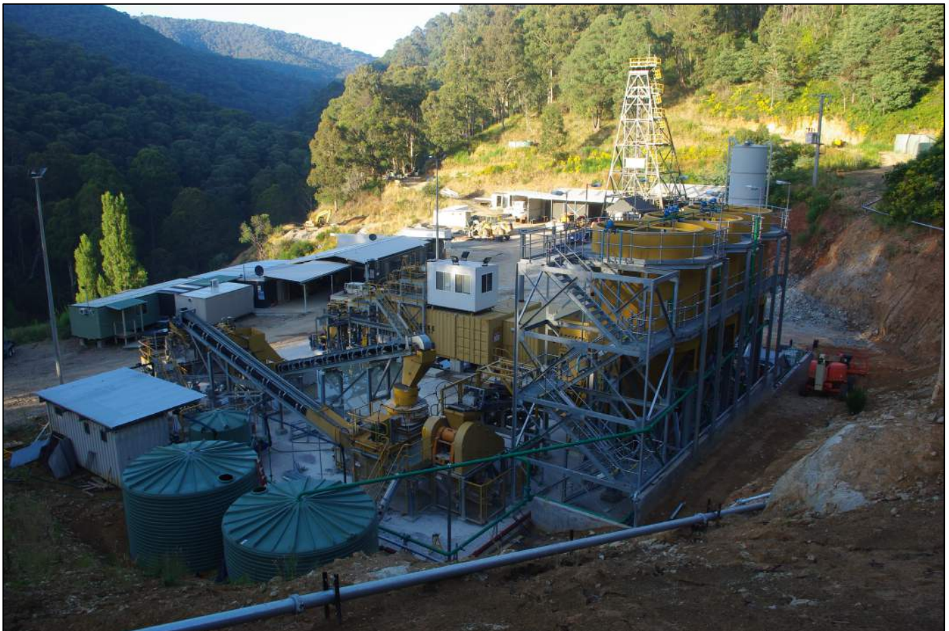
Picture 1: Morning Star processing plant, paste backfill plant, winder headframe, and mine offices.
