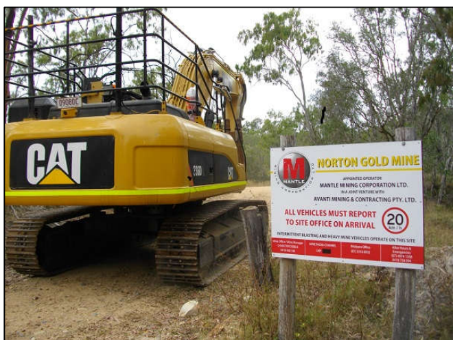
Picture 1: Mobilising to site.
